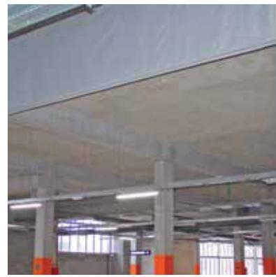
**PERLIWOOL® TERMIC** is a new concept in sprayed mortars, using rock wool as a base, mainly used for thermal insulation in construction systems.
